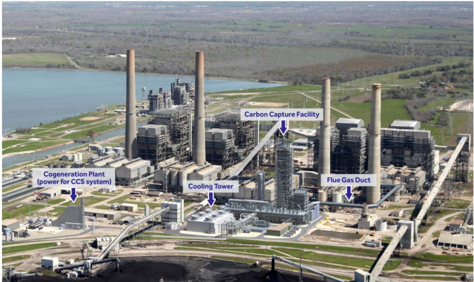
Petra Nova Power Plant, Houston, Texas (2016)
